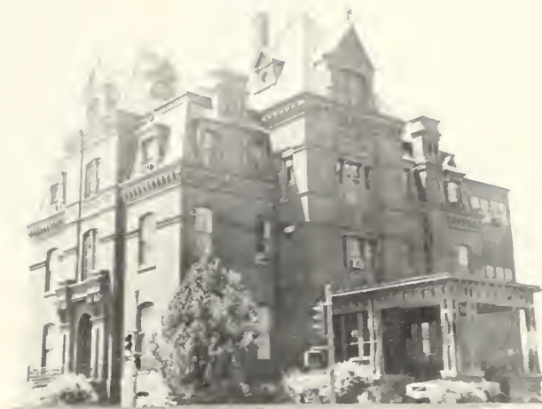
First REA headquarters was former mansion of James G. Blaine and of George Westinghouse, Jr.
